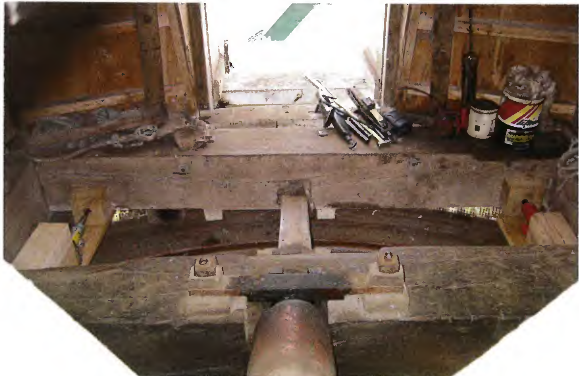
The jacks in place behind the tail beam
