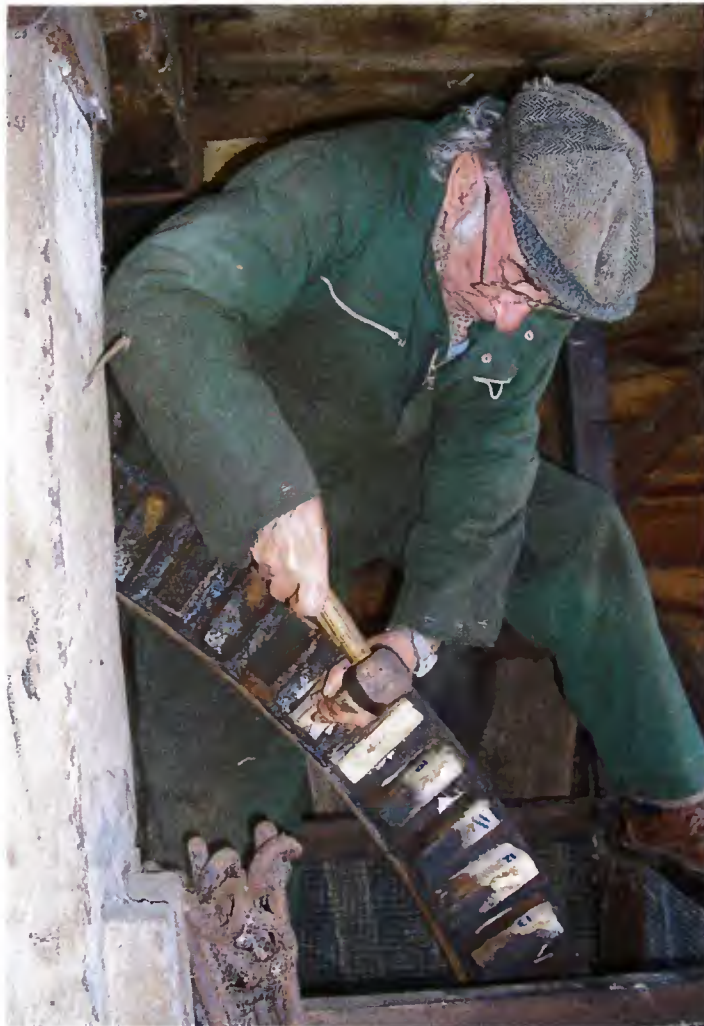
Fitting the repaired cogs. The light areas are resin repairs.
