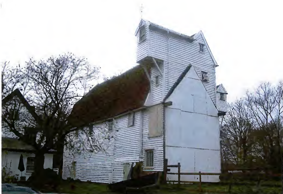
Bures mill in November 2008. The cut-off end of the late 16th century range is clearly visible.
