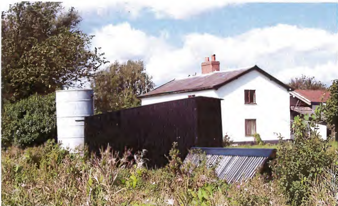
The re-clad engine shed. The low structure to the right covers some of the major buck timbers. The barn is just visible to the right of the house. (1st September 2008)
