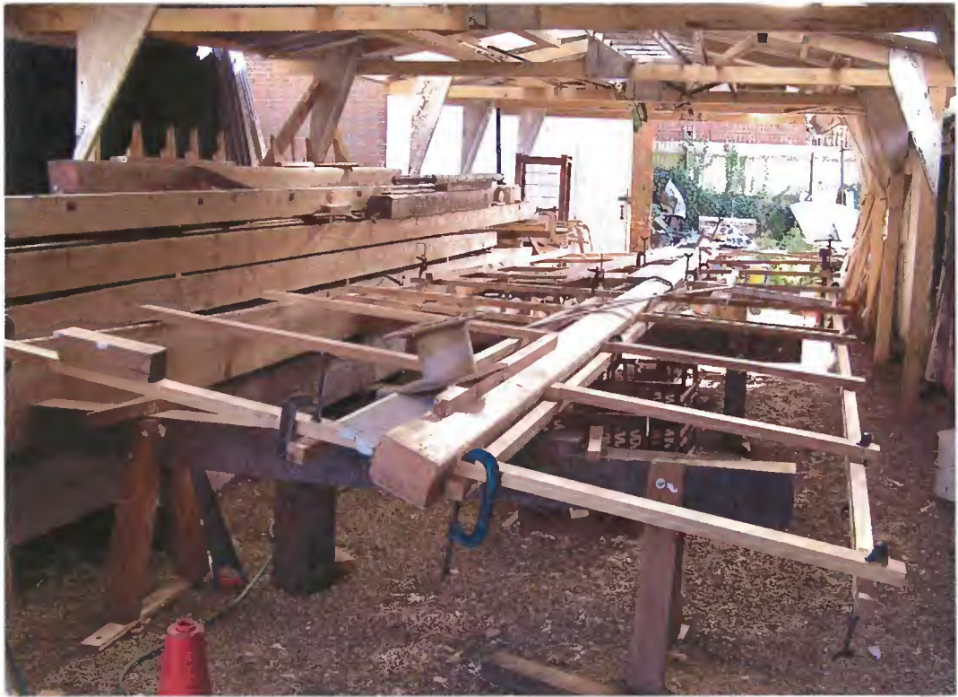
The new sails under construction at Bardwell mill
