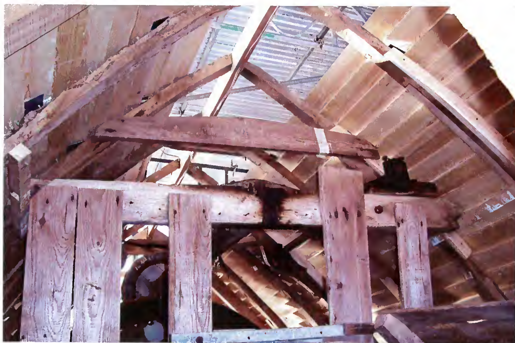
The roof of Drinkstone post mill from the tail, with new boarding & reinstated sack-hoist (February 14th 2006)
