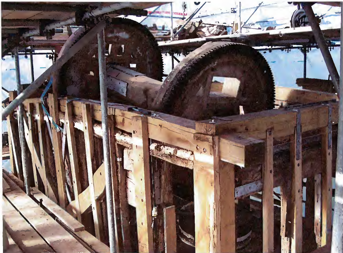
The repaired buck frame at Drinkstone
