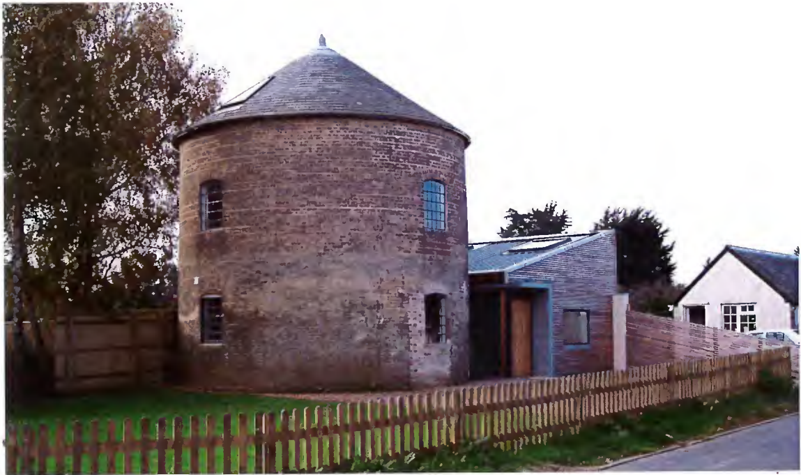
The converted roundhouse at Saxmundham
