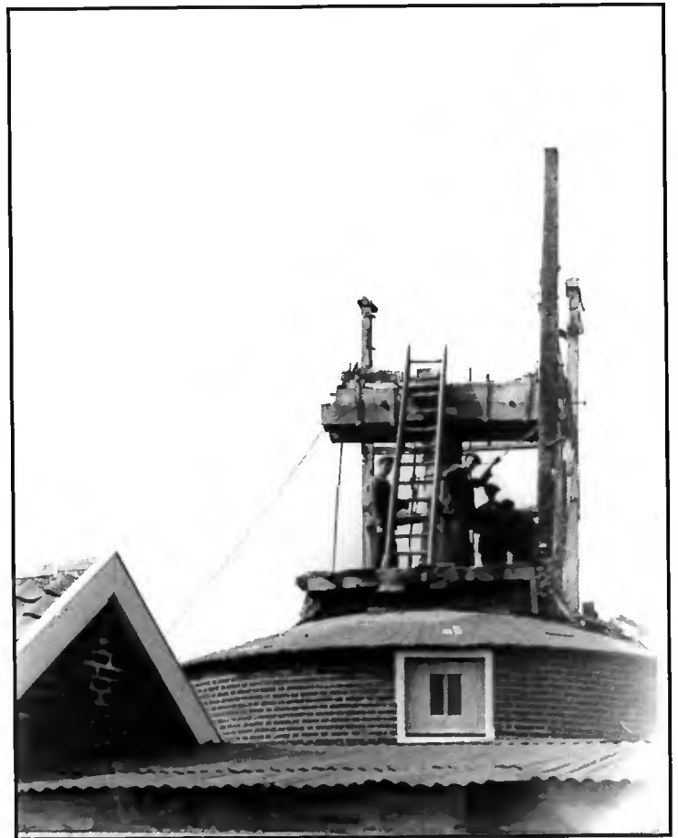
Demolition in progress in 1935
