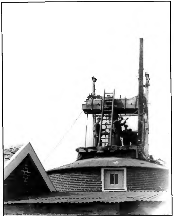
Demolition in progress in 1935
