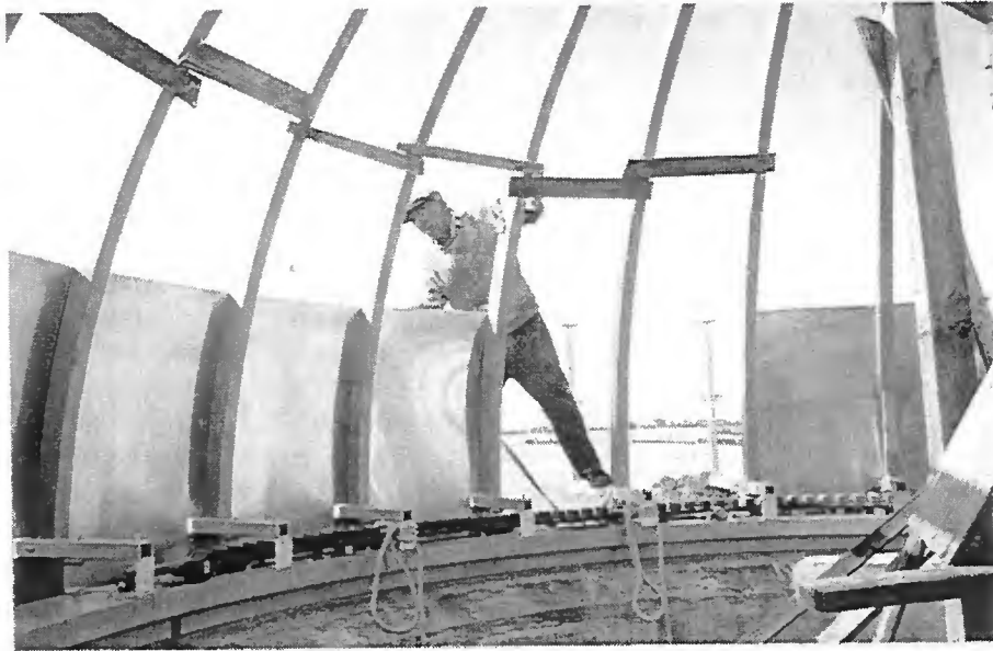
Fitting the lowest tier of aluminium sheets
