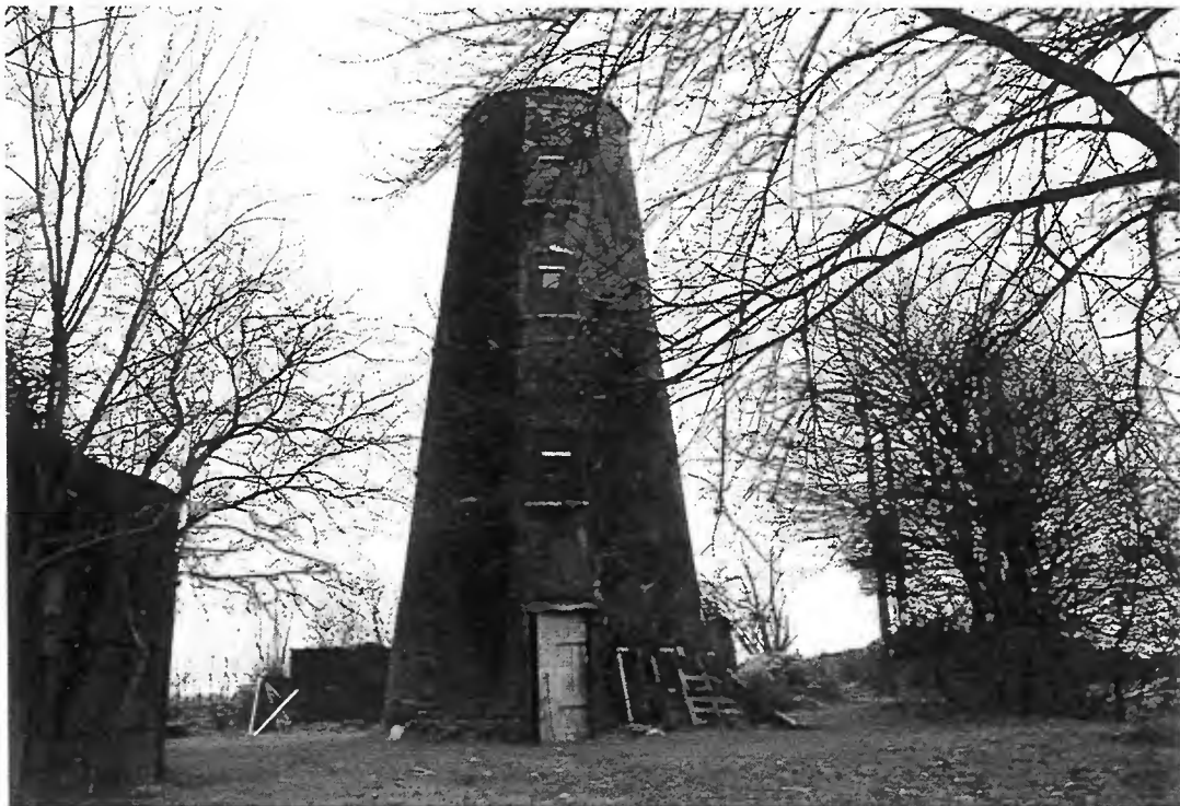
Rattlesden mill after completion of the work
