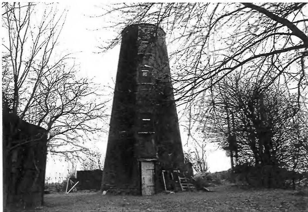
Rattlesden mill after completion of the work
