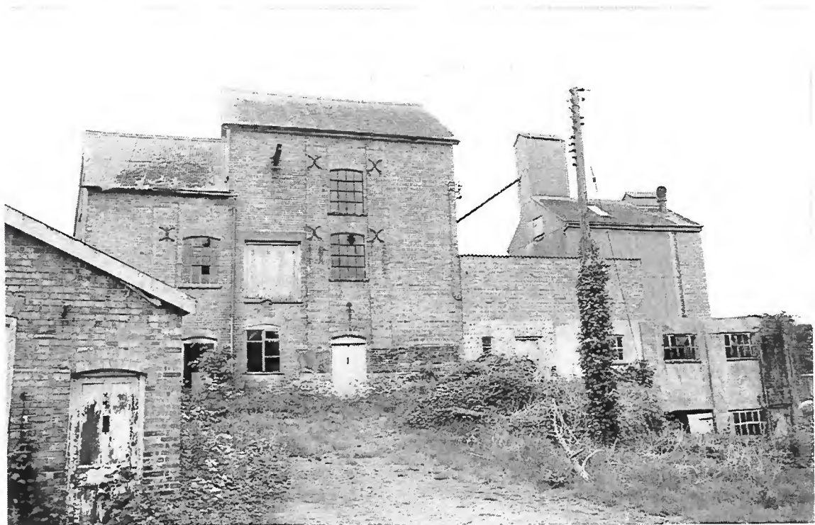
The roller mill buildings at Rattlesden. Part of the tarred smock mill base is visible each side of the door of the three-storey building
