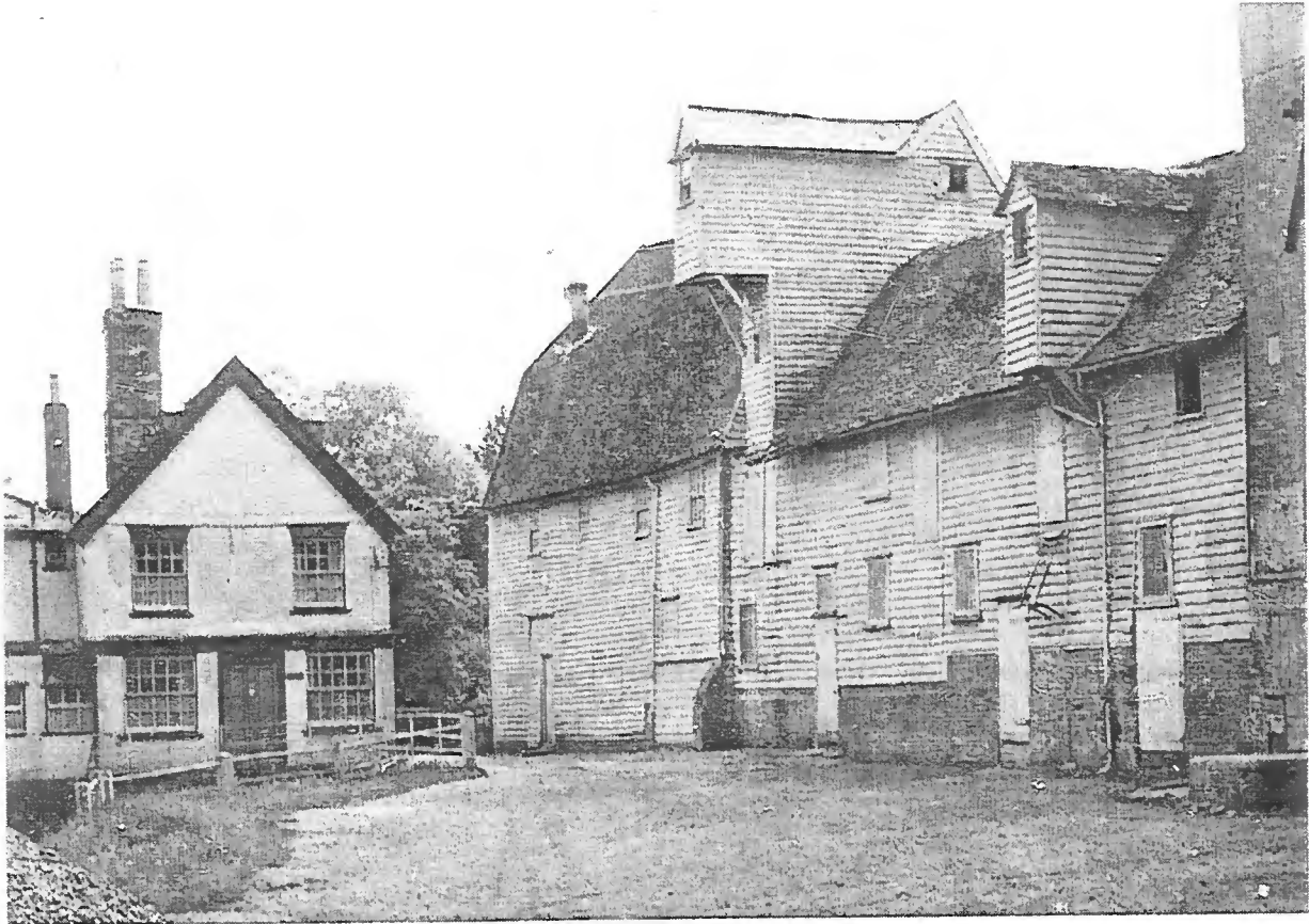
Bures Mill and Mill House from the north c.1950. The lower range nearest the camera is the Tudor mill; beyond is the 18th century addition which still stands.
