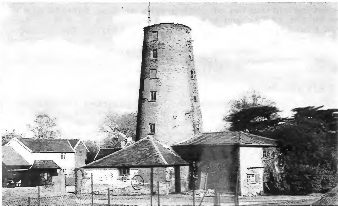
Burgh mill with attached former granary and engine shed
