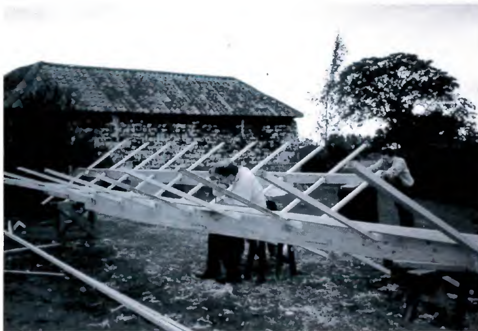
Assembly of the sail frames
