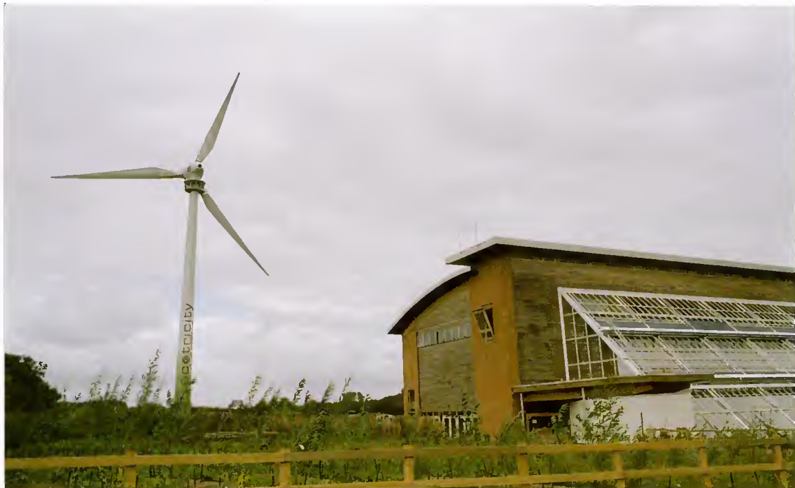
The Ecotech Centre and wind turbine
