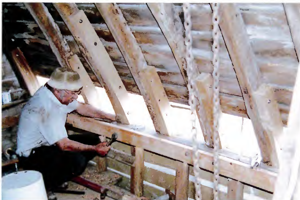
Chris Hullcoop working on repairs to the roof structure
