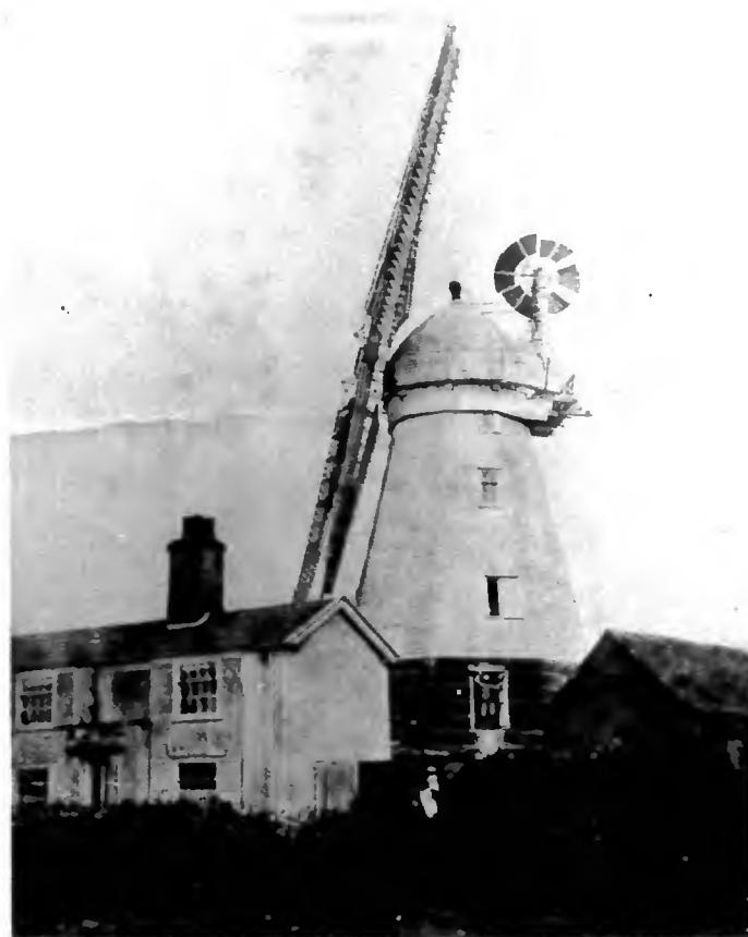
Boxford mill after 1881
