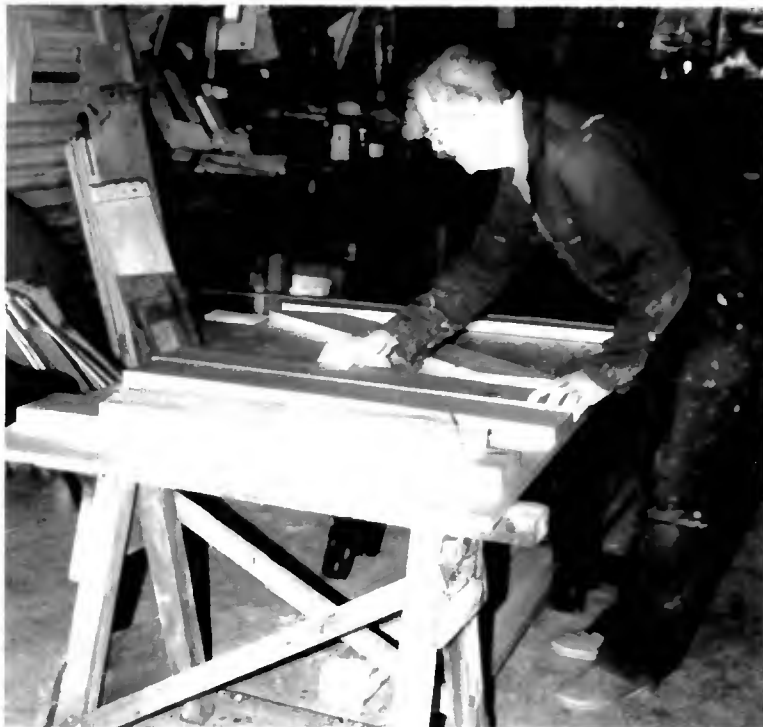
The new roundhouse door being made
