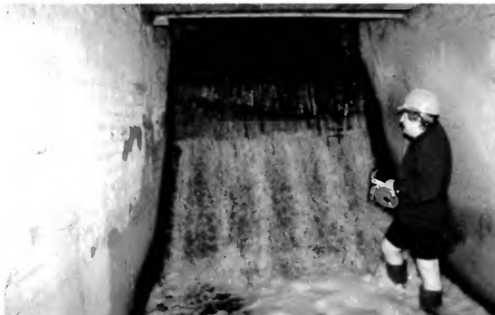
The waterwheel position at Nayland mill
