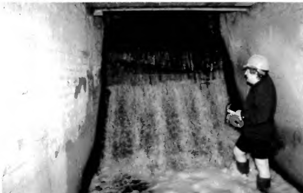
The waterwheel position at Nayland mill
