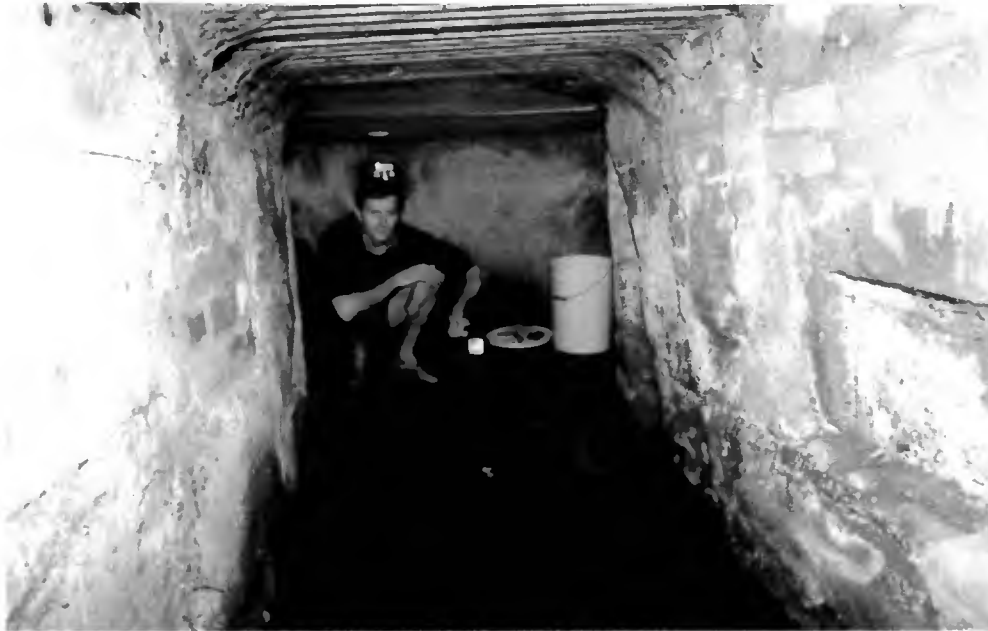
The wheel culvert under Flatford Mill
