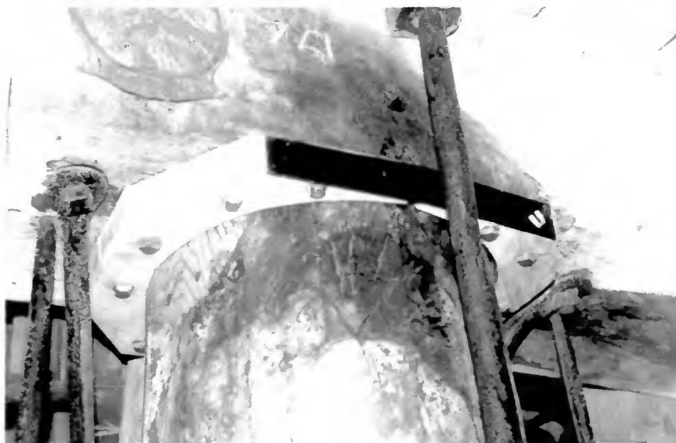
The new collar under the crowntree and patch on the post
