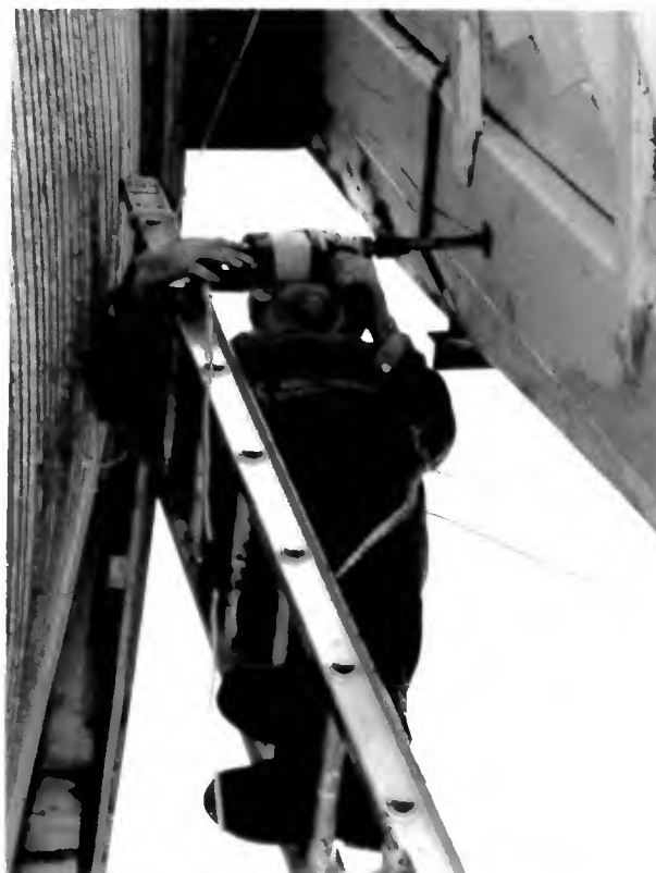
Drilling out the sailbolts
