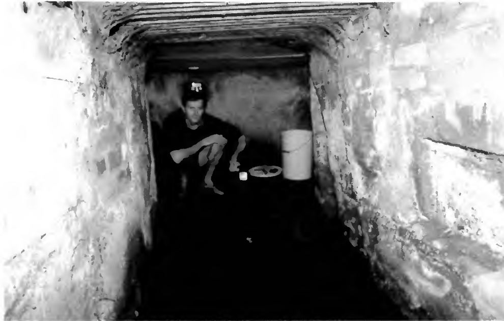
The wheel culvert under Flatford Mill
