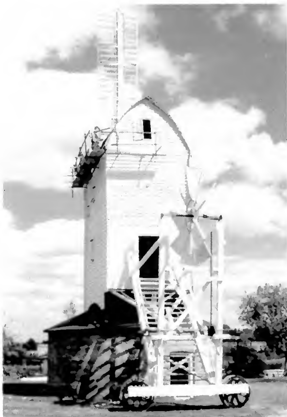
Setting up the scaffold for future work on the roof
