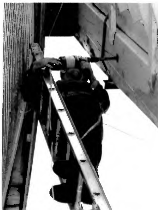
Drilling out the sailbolts
