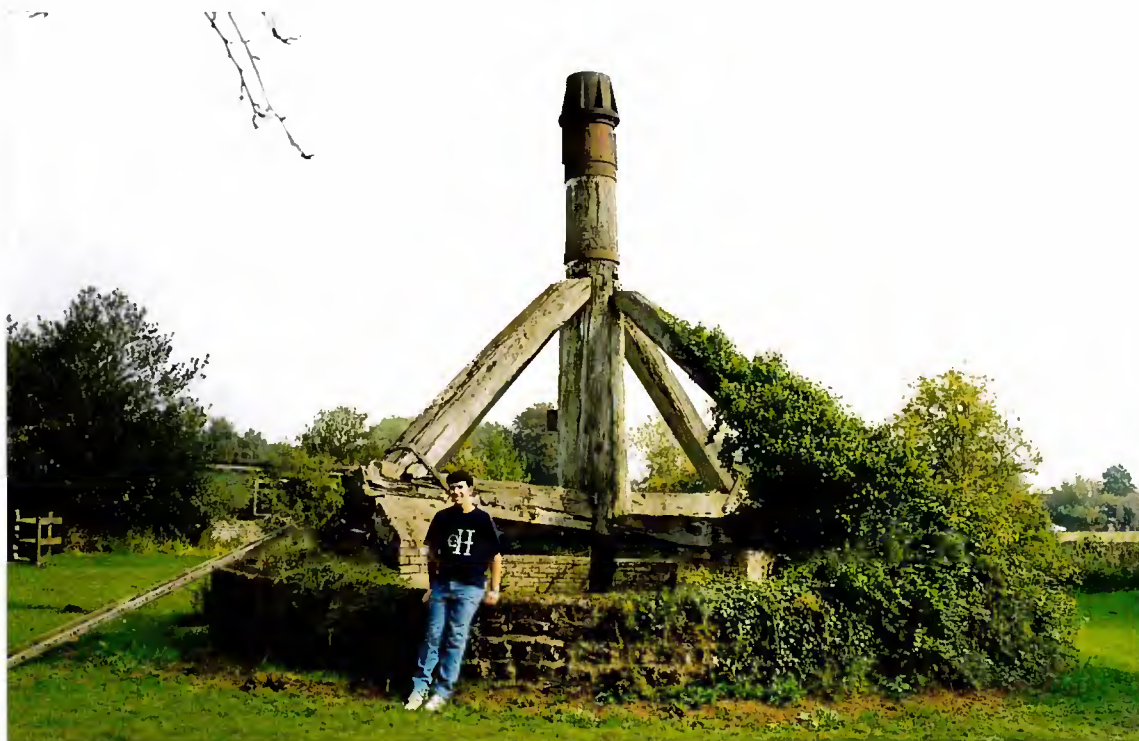
The trestle of Tottenhill mill (September 1998)
