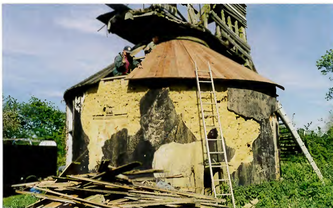
Fitting the new boards to the roundhouse roof at Syleham
