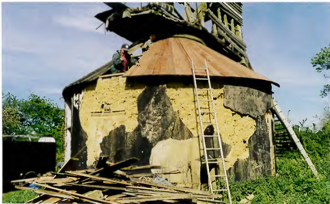
Fitting the new boards to the roundhouse roof at Syleham
