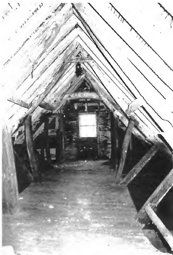
The attic walkway (1979)
