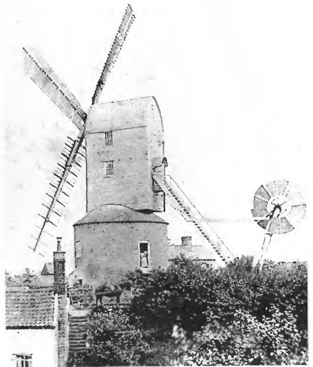
Saxmundham mill in its prime. The mill house on the left is set well below the mill, and was reached by a flight of steps, also visible.
