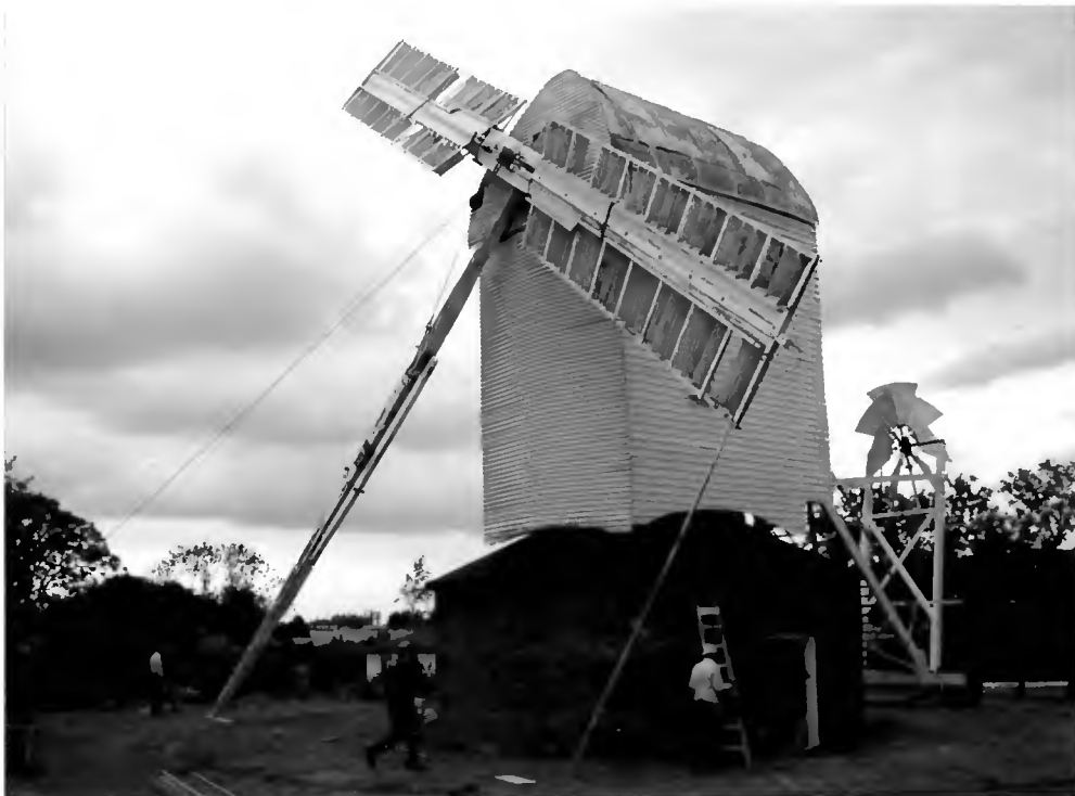
Removing the rotten sail stock
