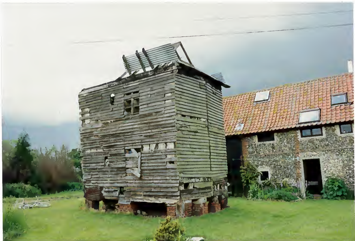
The buck, with last fragments of dovecote roof (June 1991)
