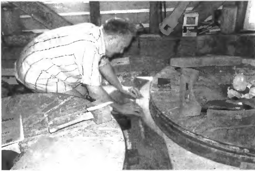
Work on the stone curbing
