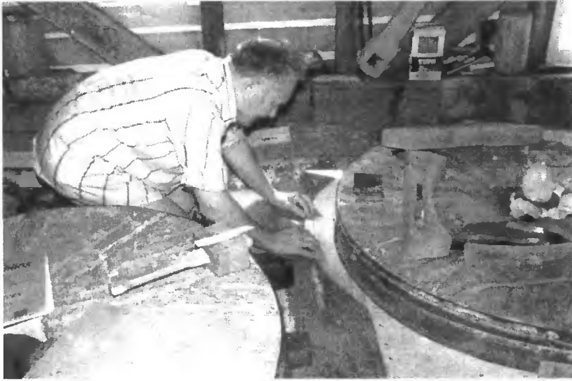
Work on the stone curbing
