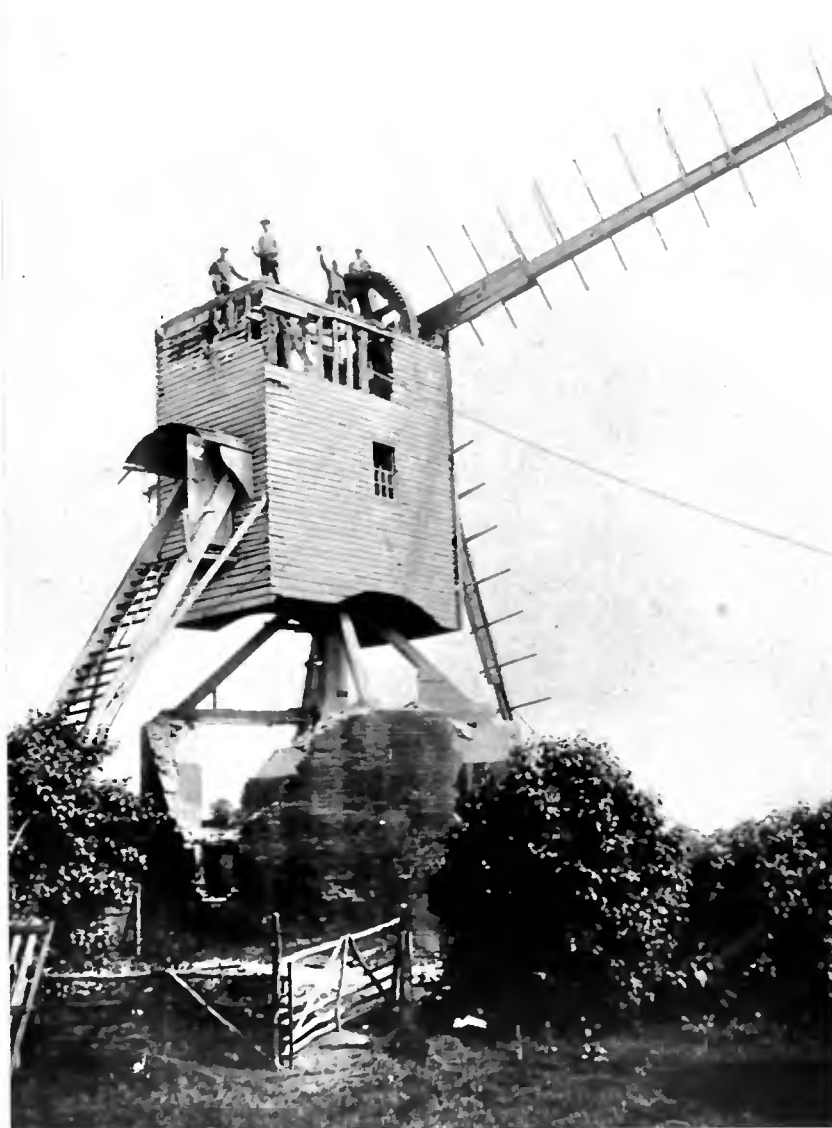
Coddenham post mill during demolition (1909)
