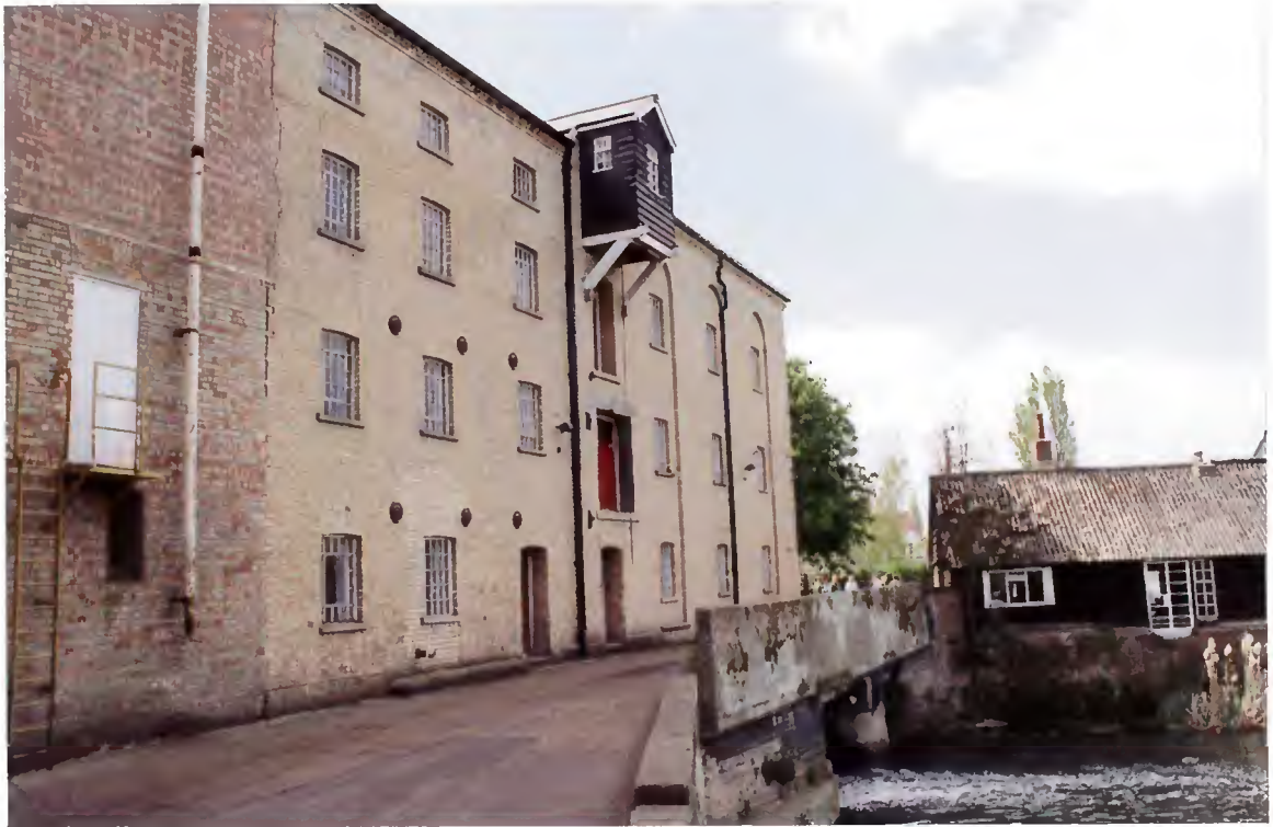
The restored flour mill
