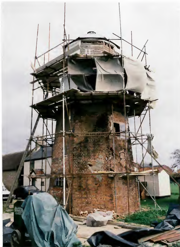
The mill during re-boarding
