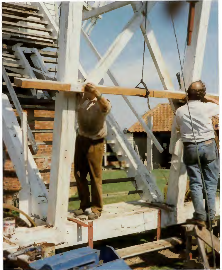
Fitting the new timber bearer on the fly posts (August 1996)
