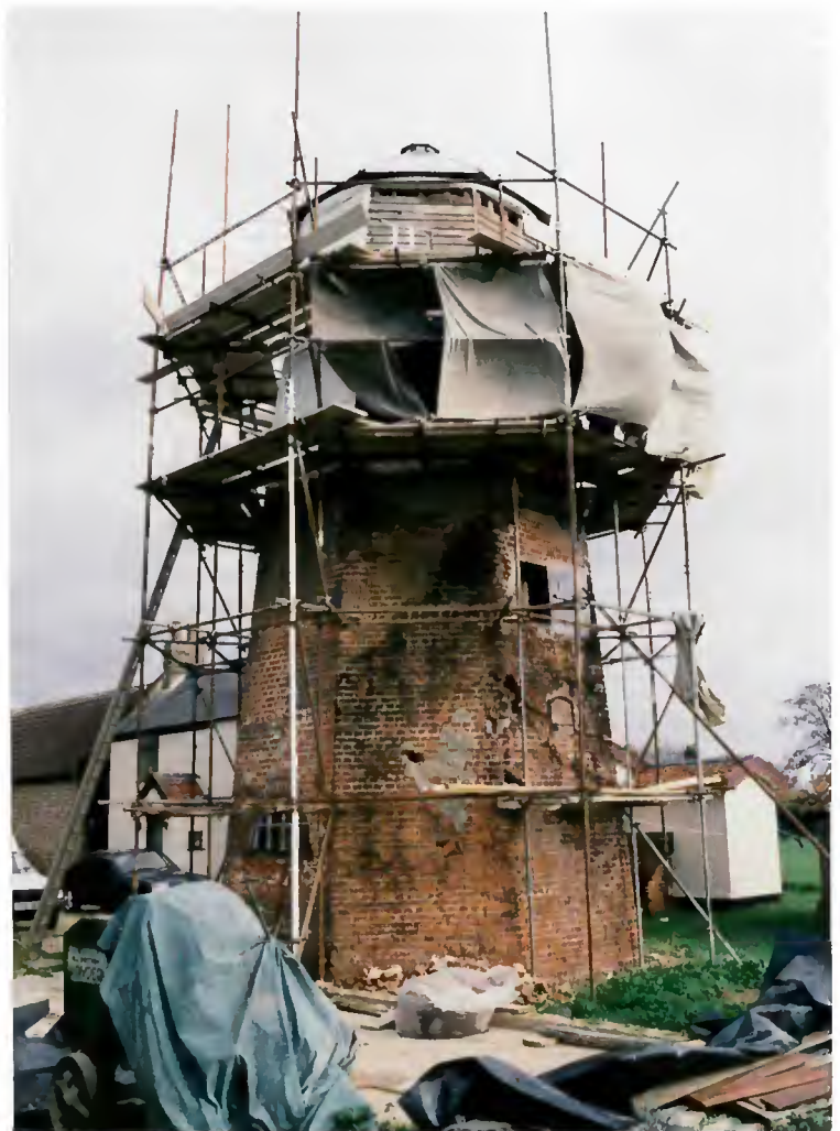
The mill during re-boarding
