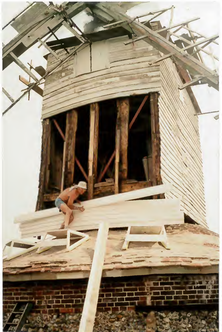
Fitting the first head boards
