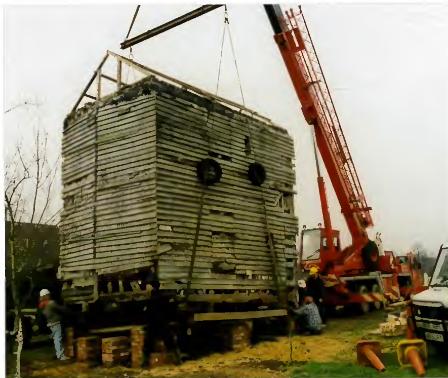
Lowering the buck onto its new site
