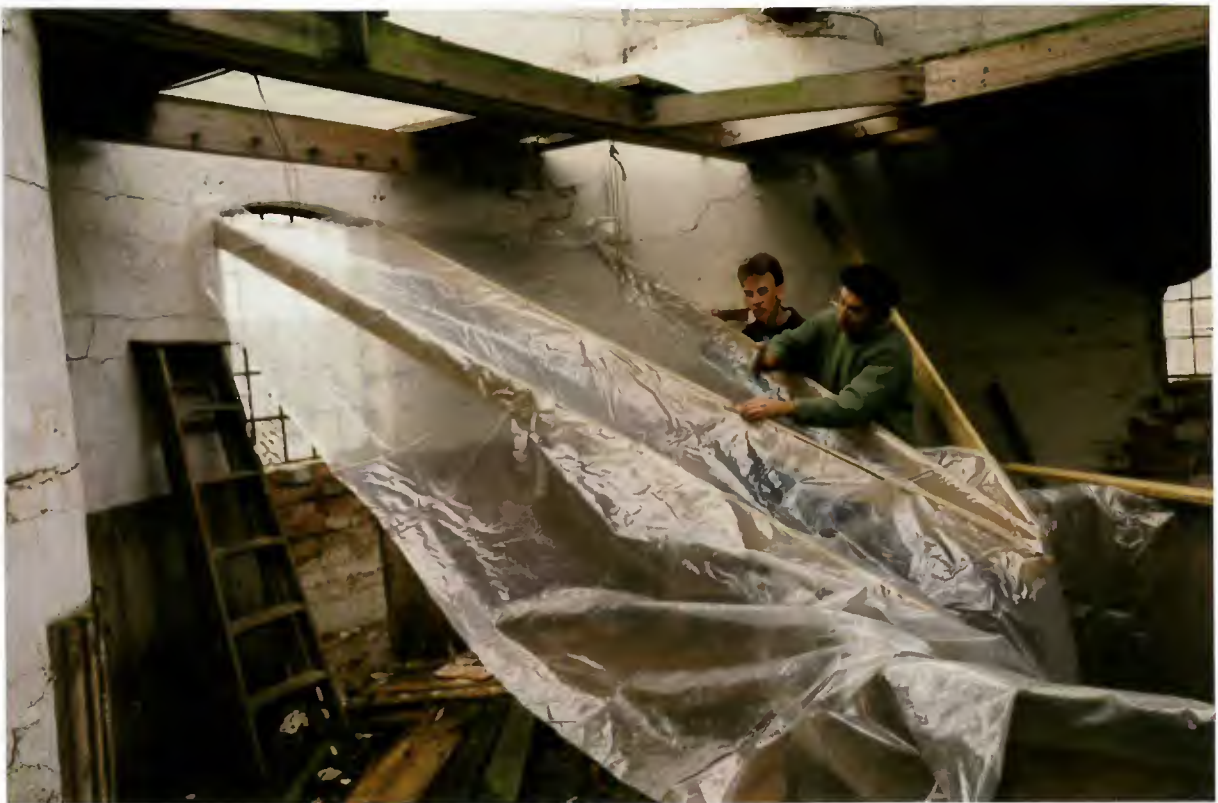
The start of the weatherproofing operation
