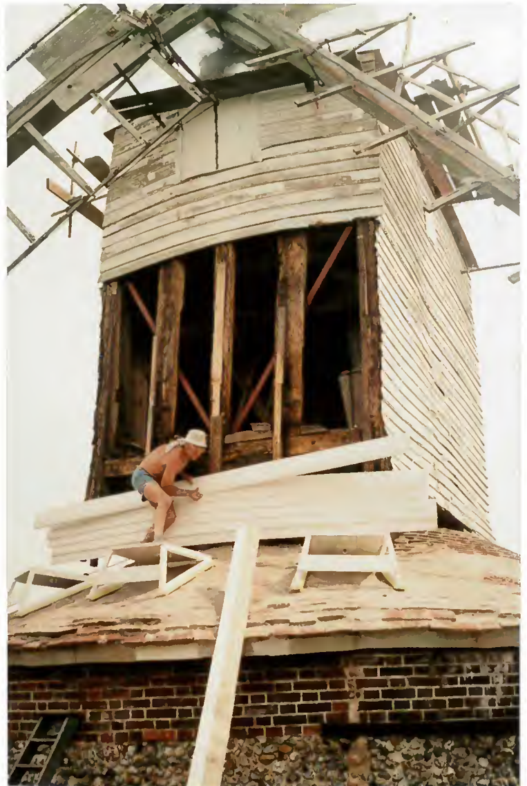
Fitting the first head boards
