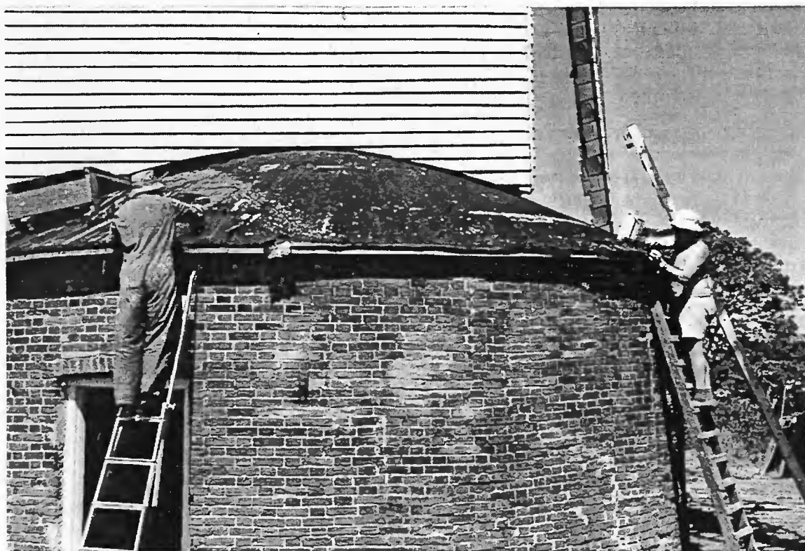
Work under way on the roundhouse roof
