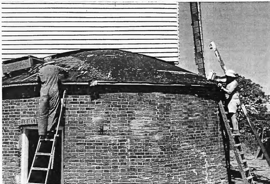
Work under way on the roundhouse roof
