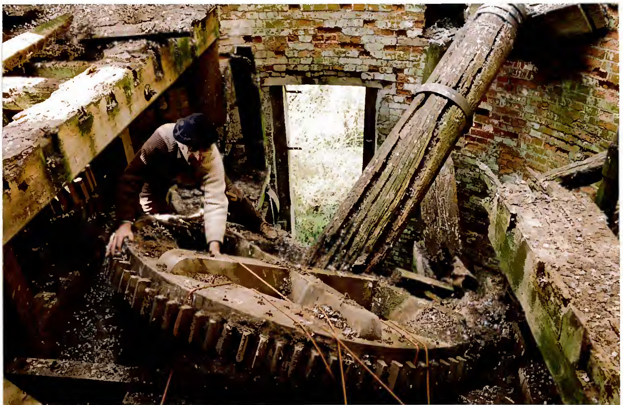
Securing the spurwheel before lowering the upright shaft
