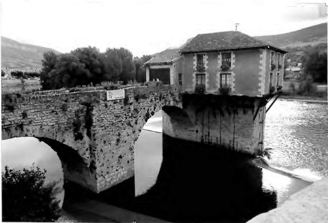
The moulin pendant on the Tarn at Millau
