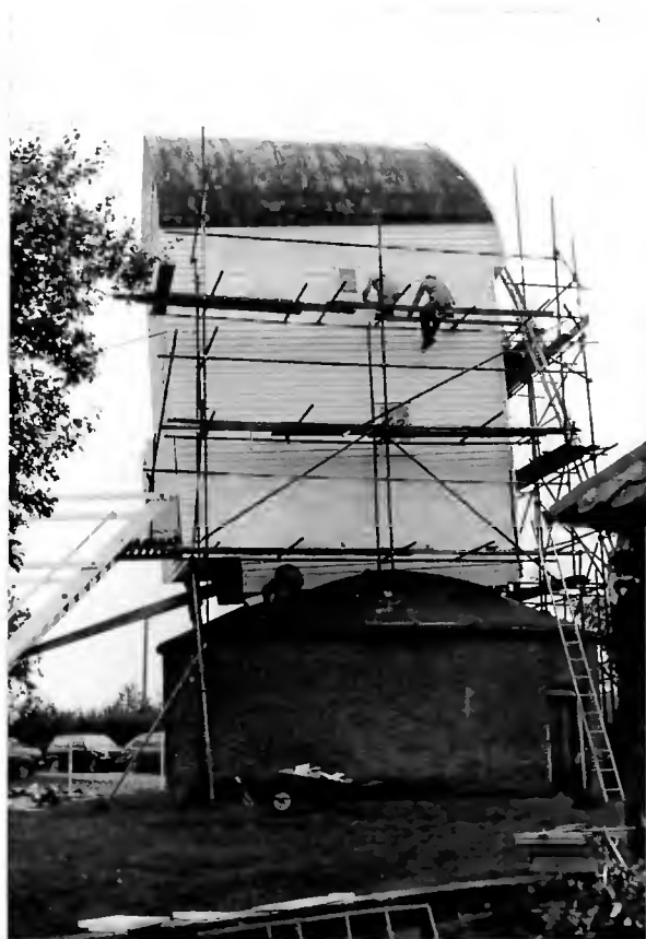
Fitting the petticoat and painting on the last weekend
