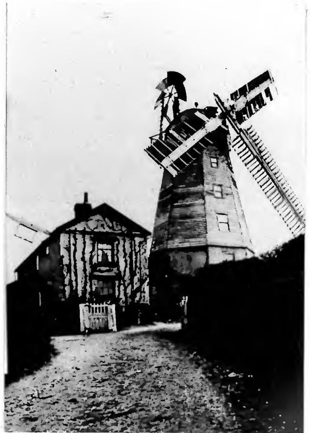
Hadleigh smock mill after gale damage, 1910. Note sail in roof!
