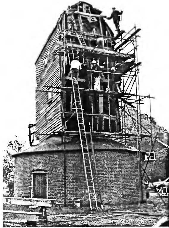
With the boards off, the frame can be examined
