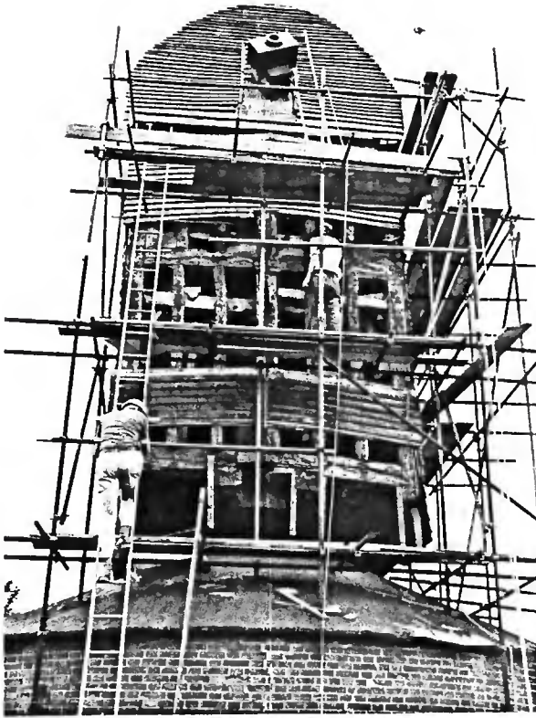
Start of the work-in: stripping boards from the head
