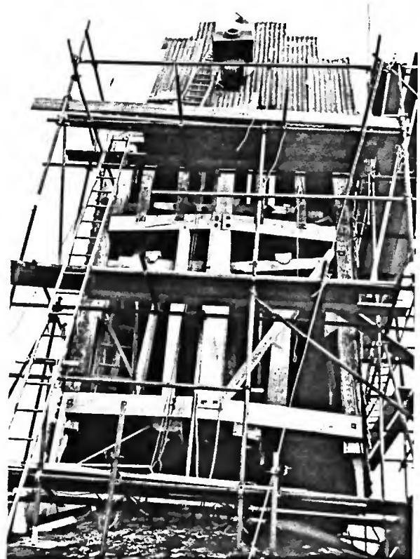
The head frame at the end of the first week's work
