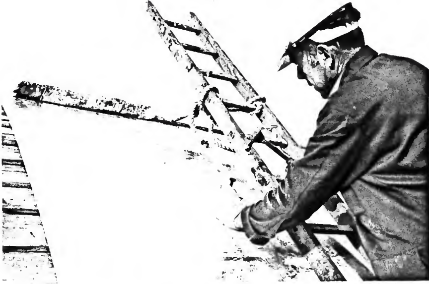
Left: Roger Skinner fixing a galvanised steel sheet on the buck roof
