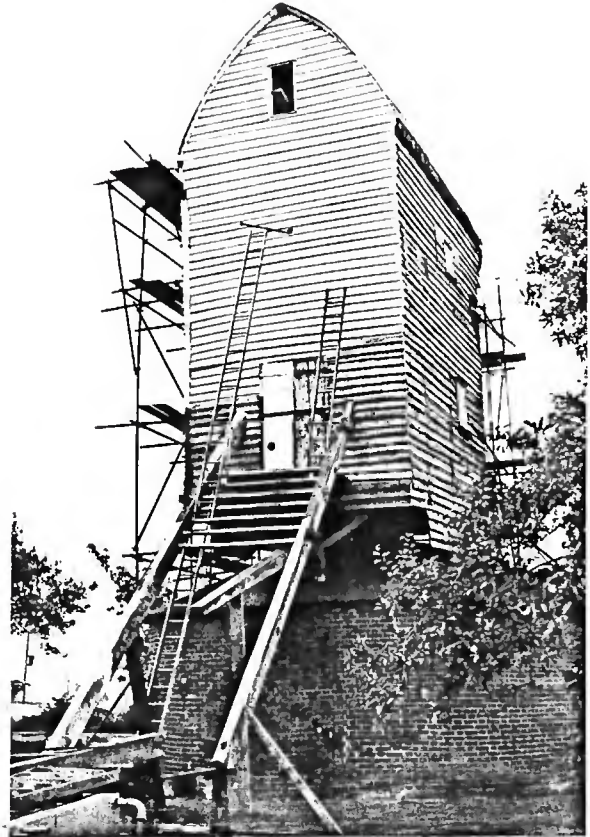
The old tail boards are re-painted
