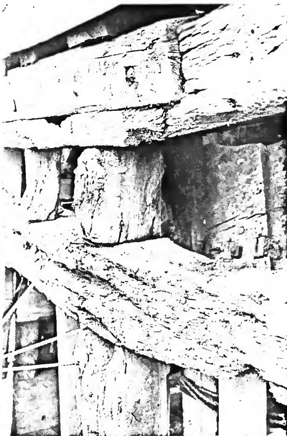
The weatherbeam (later replaced) and upper transverse beam
