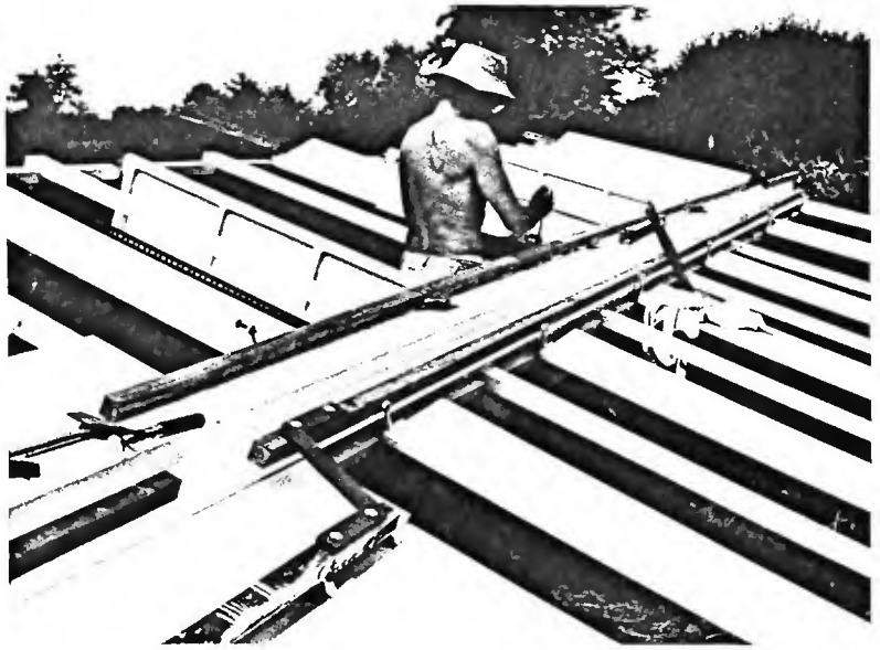
Above: Colin Budgey at work installing the sail shutters
