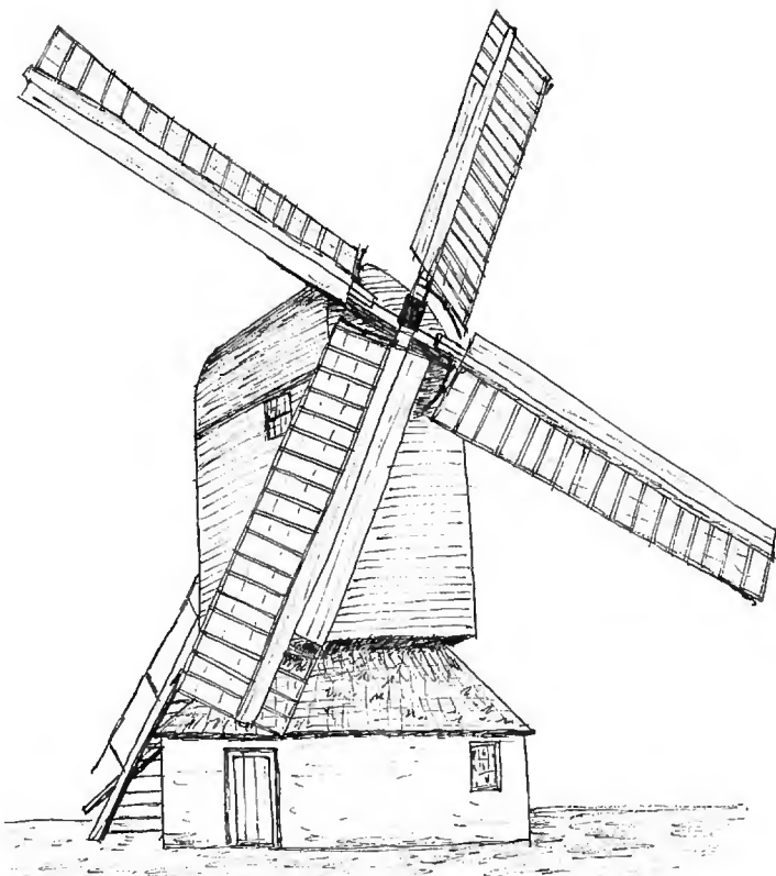
Tuddenham St. Martin mill. Spring sails with one shutter to a bay.
