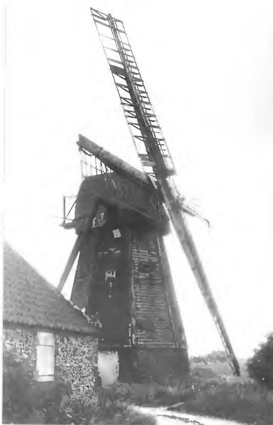
Freckenham smock mill, showing 2 common and 2 patent clockwise sails. Demolished 1967.
