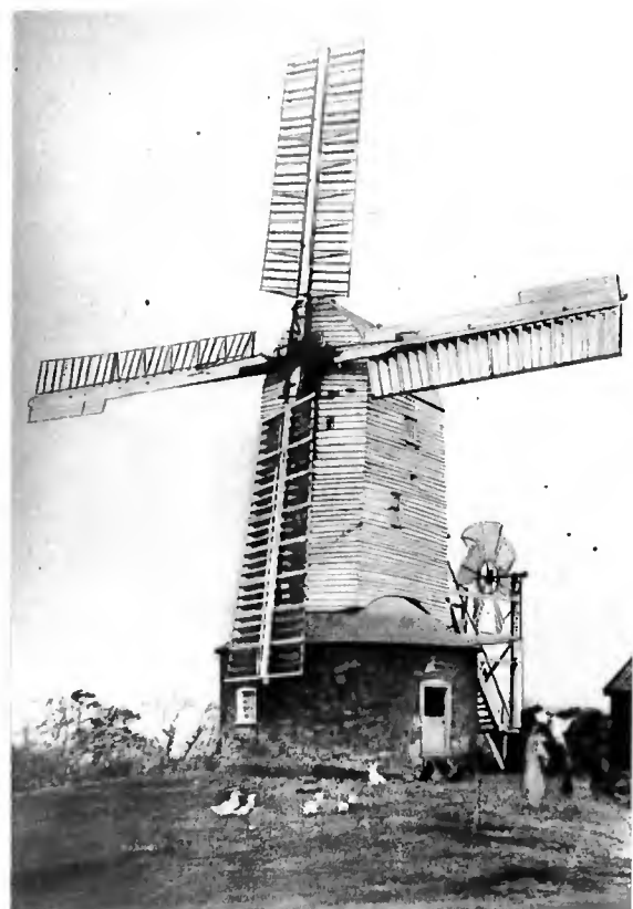
Sibton post mill, showing extra-width leading boards to one pair of sails. Demolished 1922-3.
