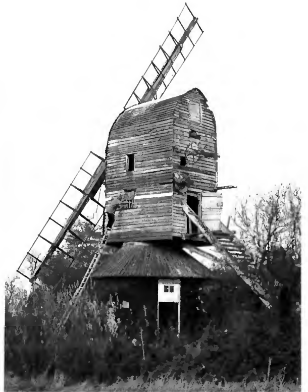
Above: Mark Barnard working on the weatherproofing of the buck windows. (Photo: Chris Hullcoop)
