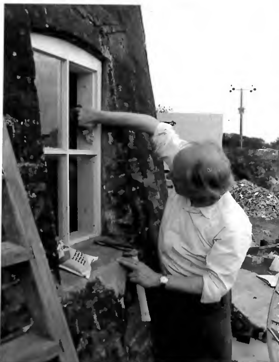
Below: Cliff Lovett glazing the new ground floor window
