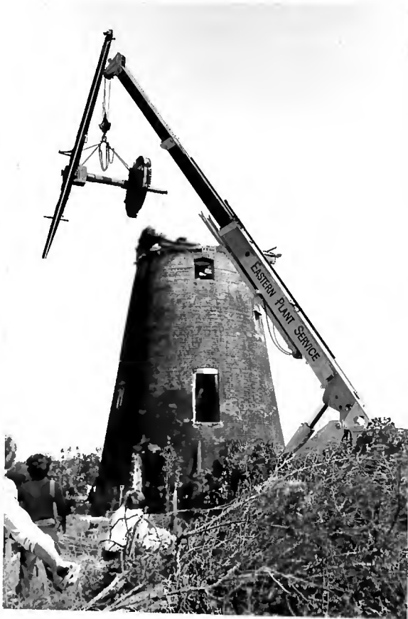
Above: lifting off the windshaft and cap frame on August 1st.
