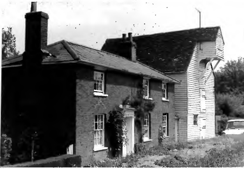
Thorrington Street Watermill
