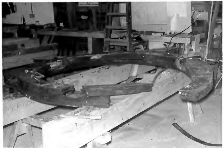
EAST BRIDGE MILL The curb being reconstructed at Jameson Marshall Ltd., Wickham Market. September 1978. (Photo: P.D.)
