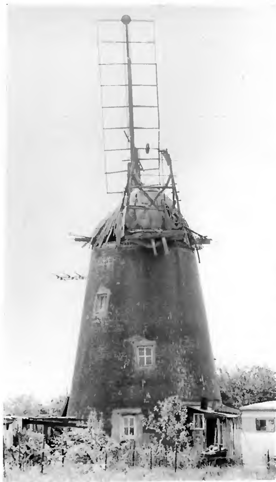
THELNETHAM MILL Taken in 1972 when the tattered remains of the cap were still in place. (Photo. by P. Dolman)
