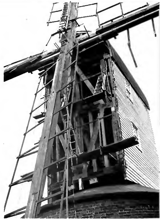
Above: New framing in the head. Picture: Mark Barnard
