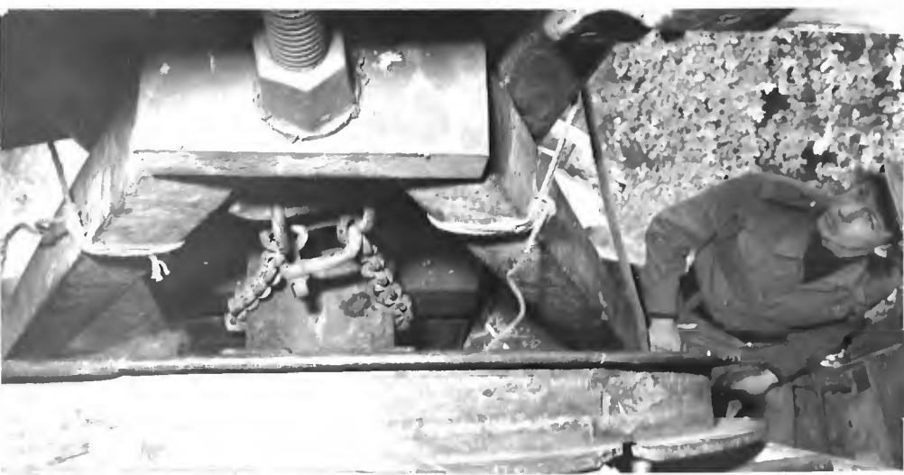
Above: Windshaft jack in use Picture: John McCann
