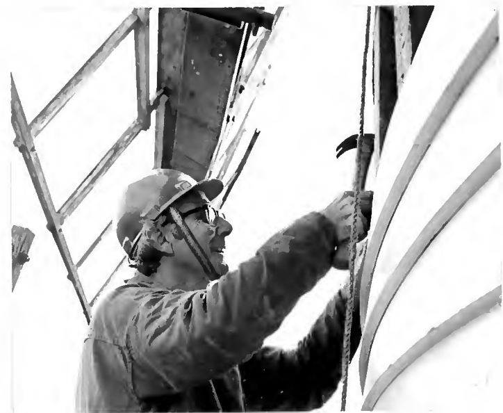
Don Porter fixing weatherboarding. Picture: John McCann
